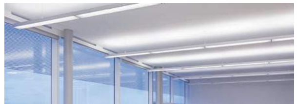
DALI buswire modules are widely used with suspended luminaires, chilled beams and busbar trunking.
