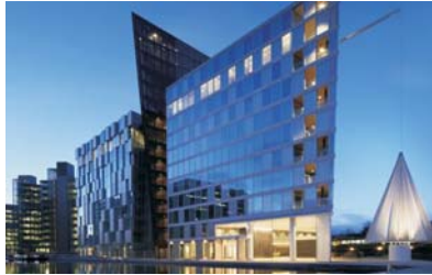
Marks & Spencer Head Office Dali buswire, Dali broadcast & circuit switching
