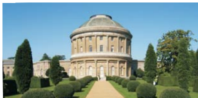
Ickworth House Dali buswire, circuit switching & dimming
