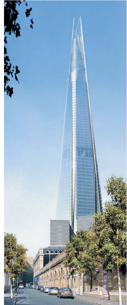
The Shard, London - Dali plug-in, broadcast & buswire, circuit switching, emergency monitoring
